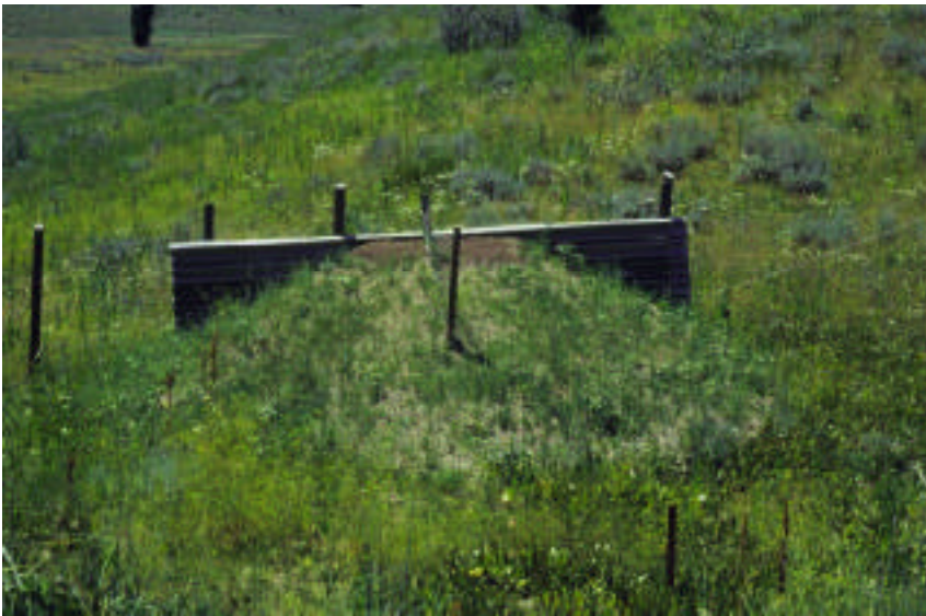
FIGURE 2 Example earthen escape ramp (19).
